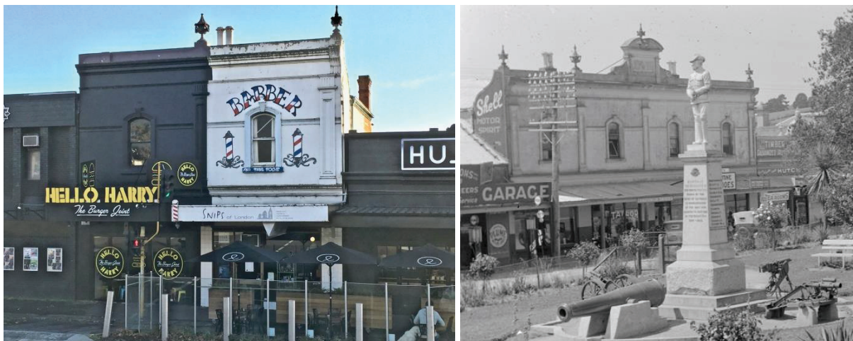
Figure 1. Contemporary image of the Poyner shops in comparison with a historical image (c.1930s) showing the previous built form and detailing. Half of the building and other detailing has been demolished, and the lower façade heavily altered.
